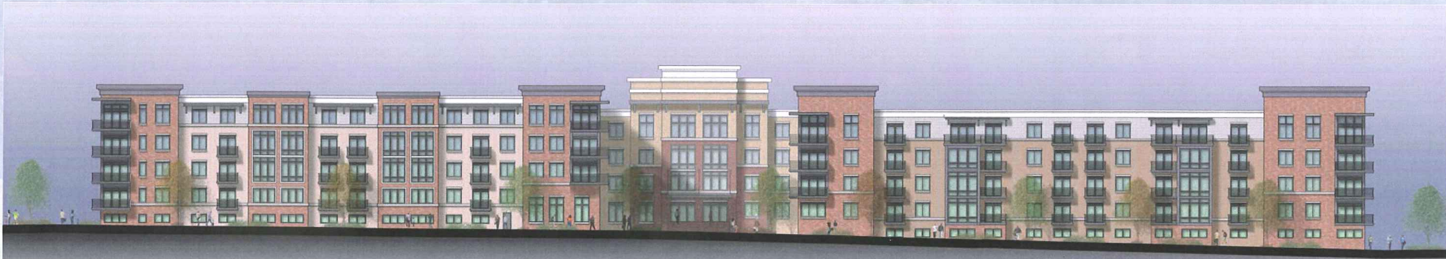
Front Elevation of Building 7
